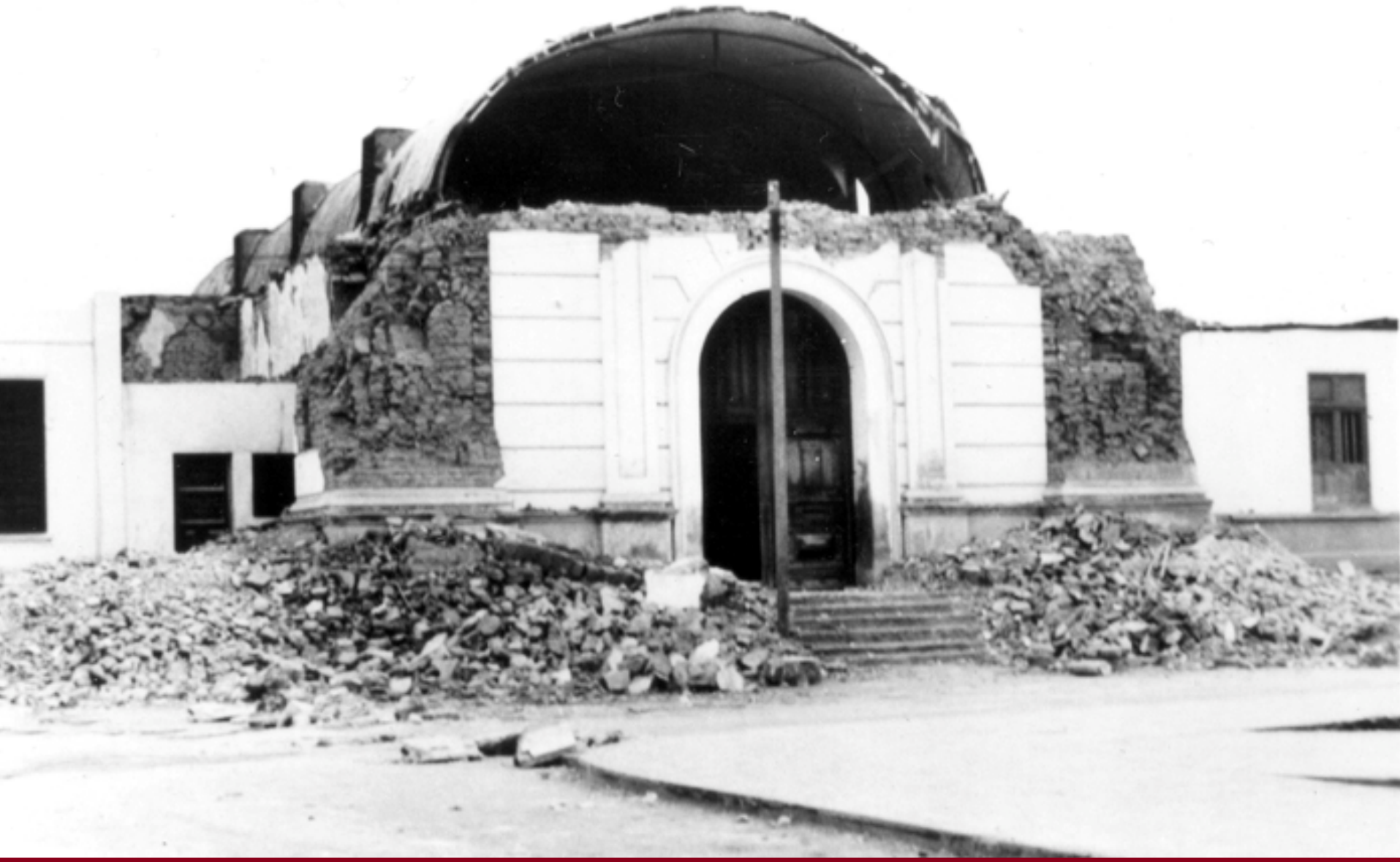
Peru Earthquake October 3, 1974. Heavily damaged building in the Lima area after the magnitude 7.6 shock. 1974. Page 11, Earthquake Information Bulletin, v.7, no.2.
