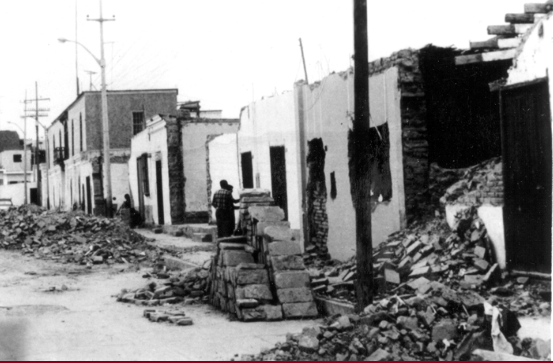
Peru Earthquake October 3, 1974. Severe damage to adobe and quincha buildings in Chorrillos District. Hundreds of families were left homeless in the aftermath of the earthquake. 1974. Page 3, Earthquake Information Bulletin, v.7, no.2. Bulletin-0007
